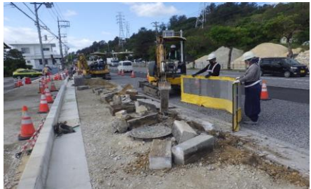
▶縁石撤去状況 2023/3
